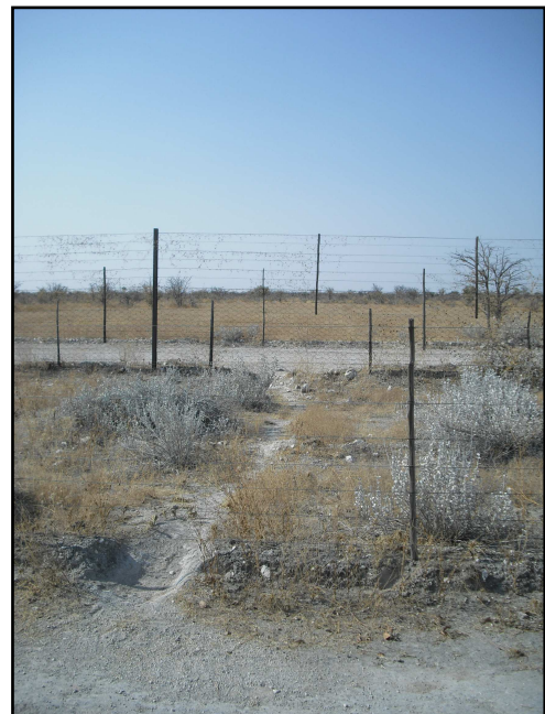
Fig. 8: The fence of the Etosha National Park is in desolate condition over large parts (A. J.)
