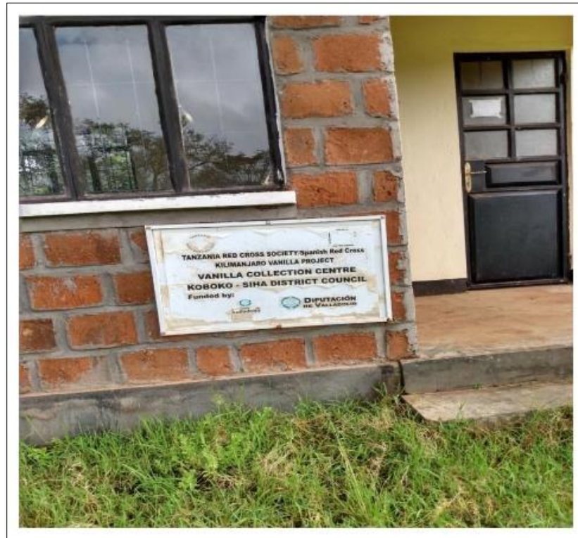
Figure 5. 5 The Vanilla Collection Centre constructed by the facilitation of Red Cross for UWAVAKI's vanilla collection
