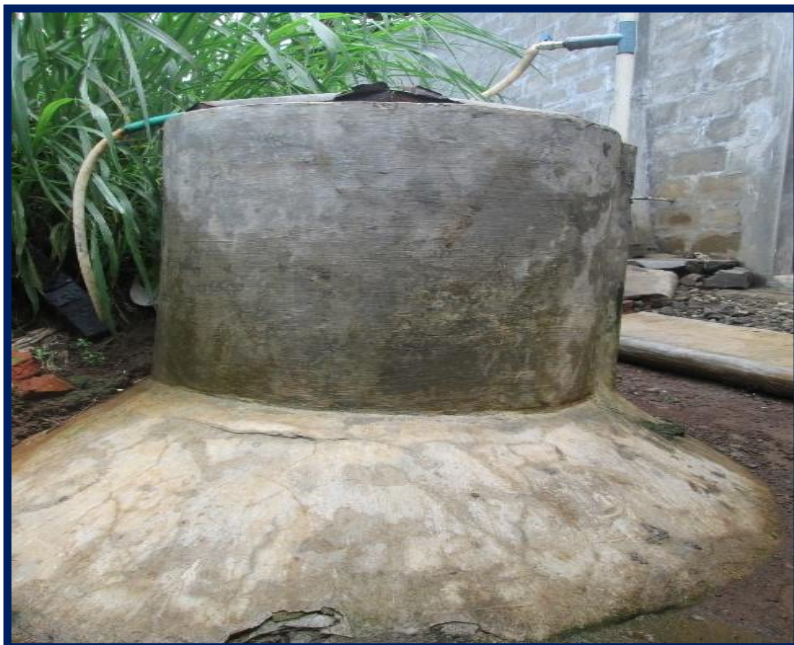
Figure 23: Fixed dome biogas reactor
