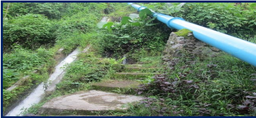
Figure 25: Penstock in WOT Lemah micro-hydro system
