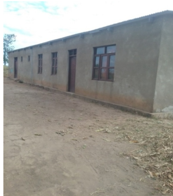
Small-scale pineapples processing facility that is built in Madeke Village
