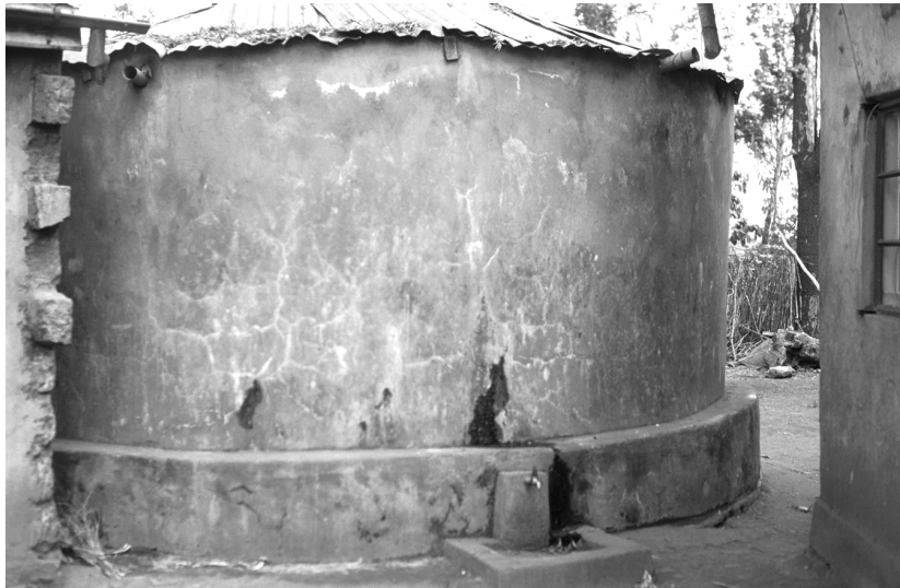
Fig. 84: Water tank on farm 1K-I
