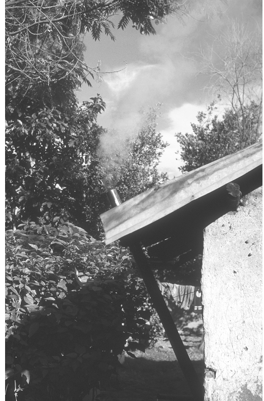
Fig. 113: Self-constructed chimney on the kitchen-roof of 2T-I
