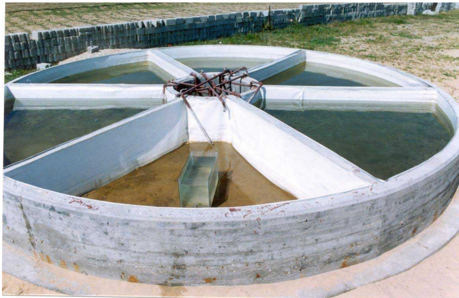
Figure 2.6b. Section pond at EPRI (Gaza). It is divided into six sections which were used for controls and contamination experiments with petroleum model compounds.
